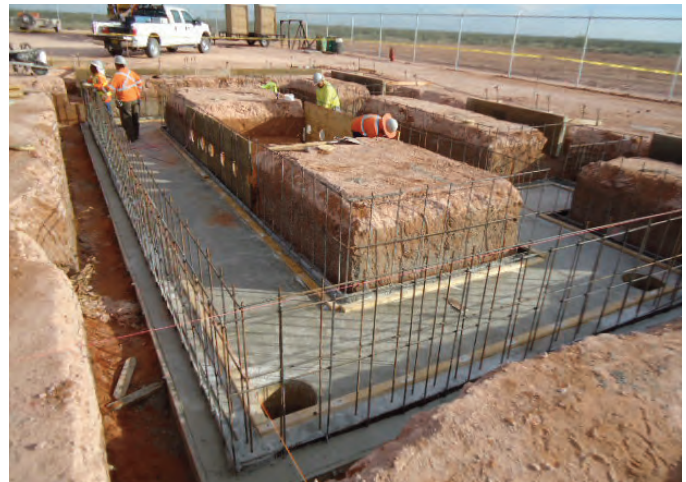
Substation work has begun on the Custer Mountain-Ponderosa 115 kV transmission line near Jal, N.M. Crews work on excavating and framing the control house that will sit at the new Ponderosa Substation about eight miles west of Jal.
