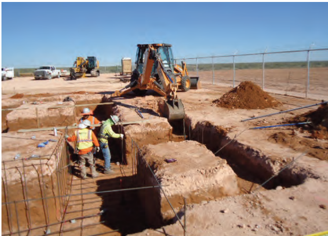
Substation work has begun on the Custer Mountain-Ponderosa 115 kV transmission line near Jal, N.M. Crews work on excavating and framing the control house that will sit at the new Ponderosa Substation about eight miles west of Jal.
