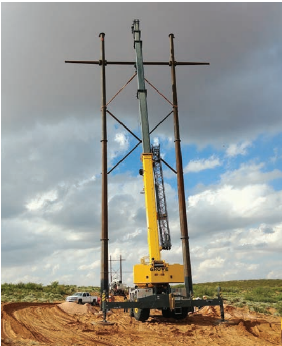
Crews are setting structures and building foundations on the Hobbs-China Draw project.
