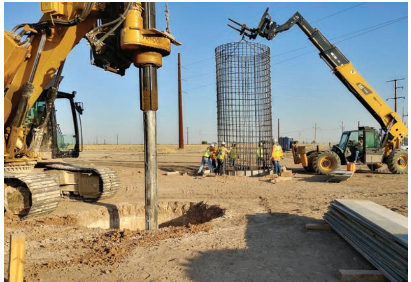
Crews are setting structures and building foundations on the Hobbs-China Draw project.
