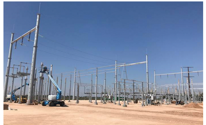
The Wolfforth Substation is being upgraded near Wolfforth, Texas.
