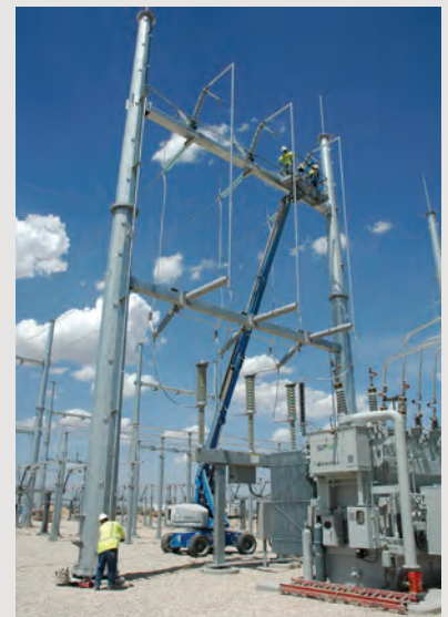
Crews work on the China Draw Substation.
