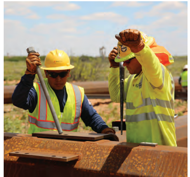
A structure is bolted together before setting west of Jal.
