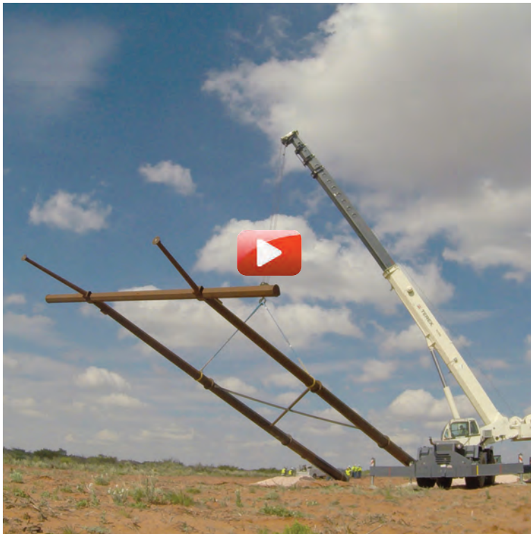
A structure is bolted together before setting west of Jal.
